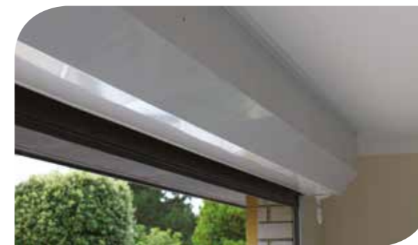
Internal view showing canopy (box)
